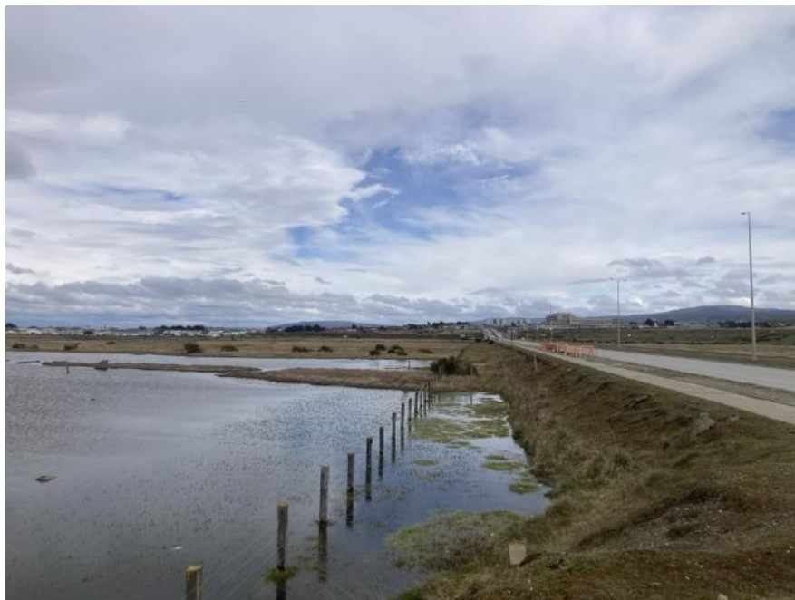
Figure 5-23: View of the Tres Puentes Wetland
