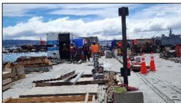
Photograph 3-1: Installation of work equipment on the dock
