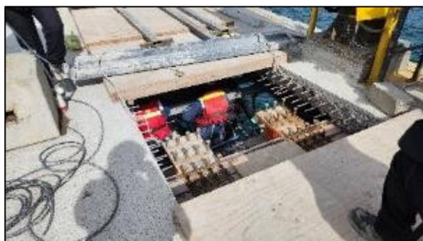
Photograph 3-3: Partial demolition of slab
