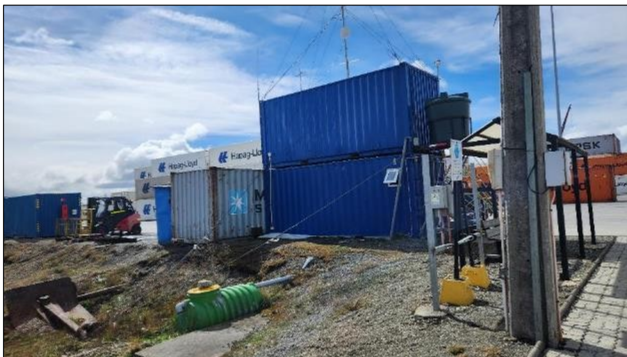
Photo 3-12: Septic tank at the Maritime Agency offices
