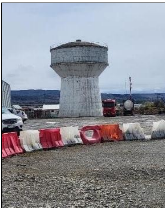
Photograph 3-6: Water intake for supplying drinking water
