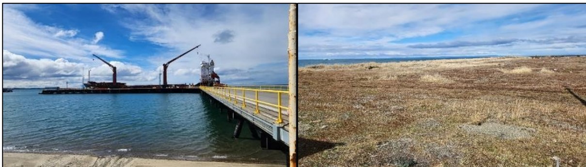
Photograph 5-3: Built-up area in the port
